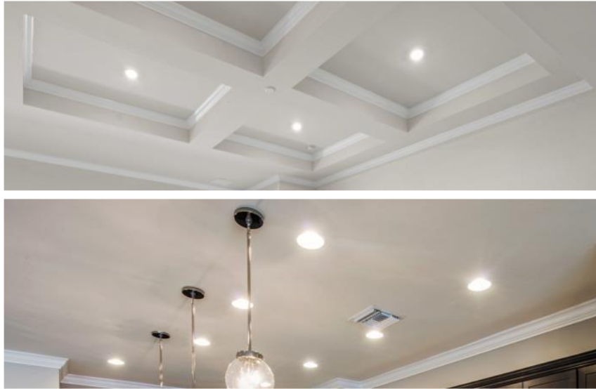
Recessed LED Lighting
